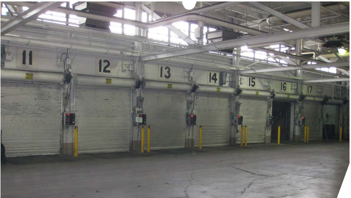
Interior view of the North side dock doors
