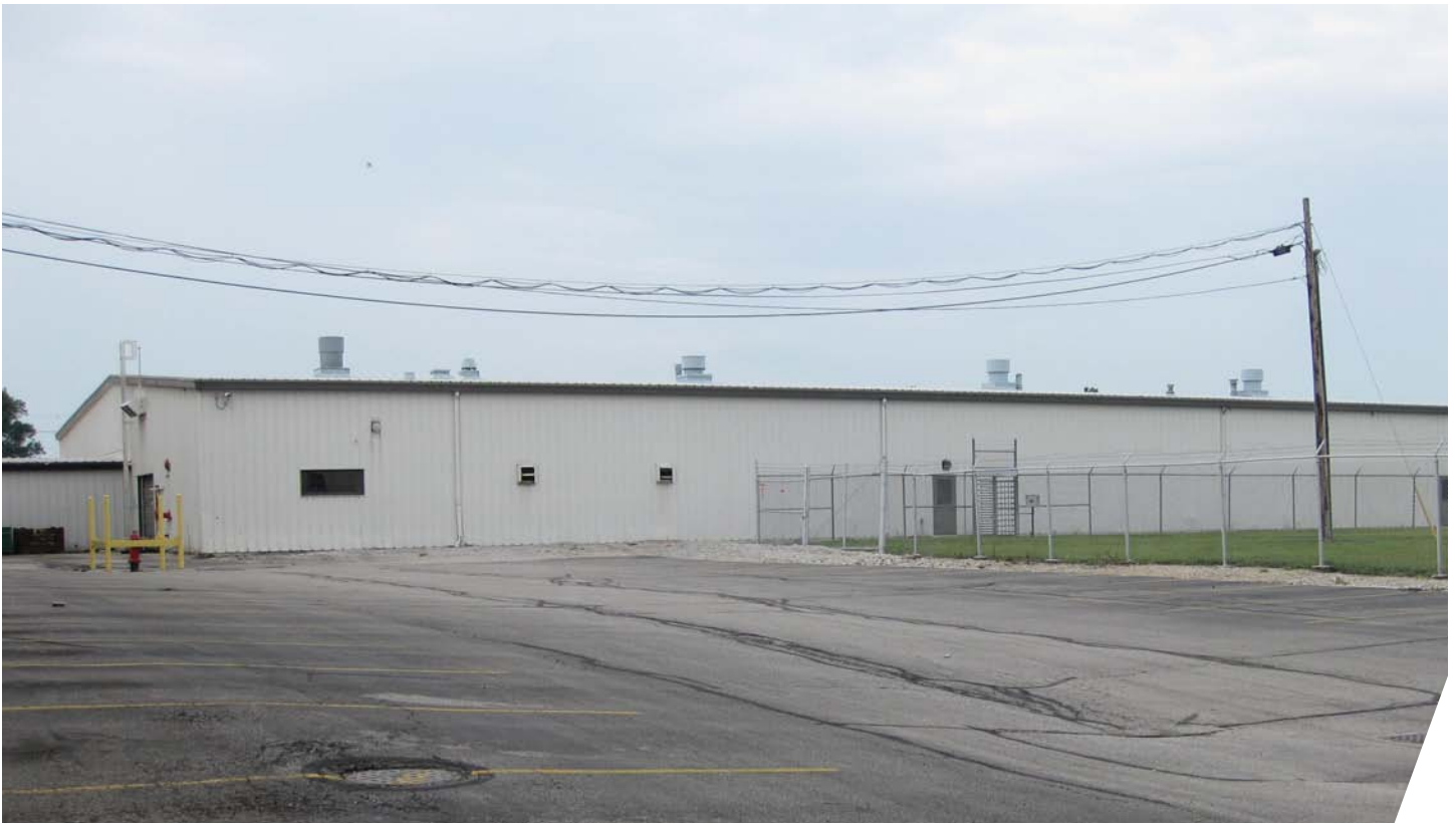
South side of warehouse
