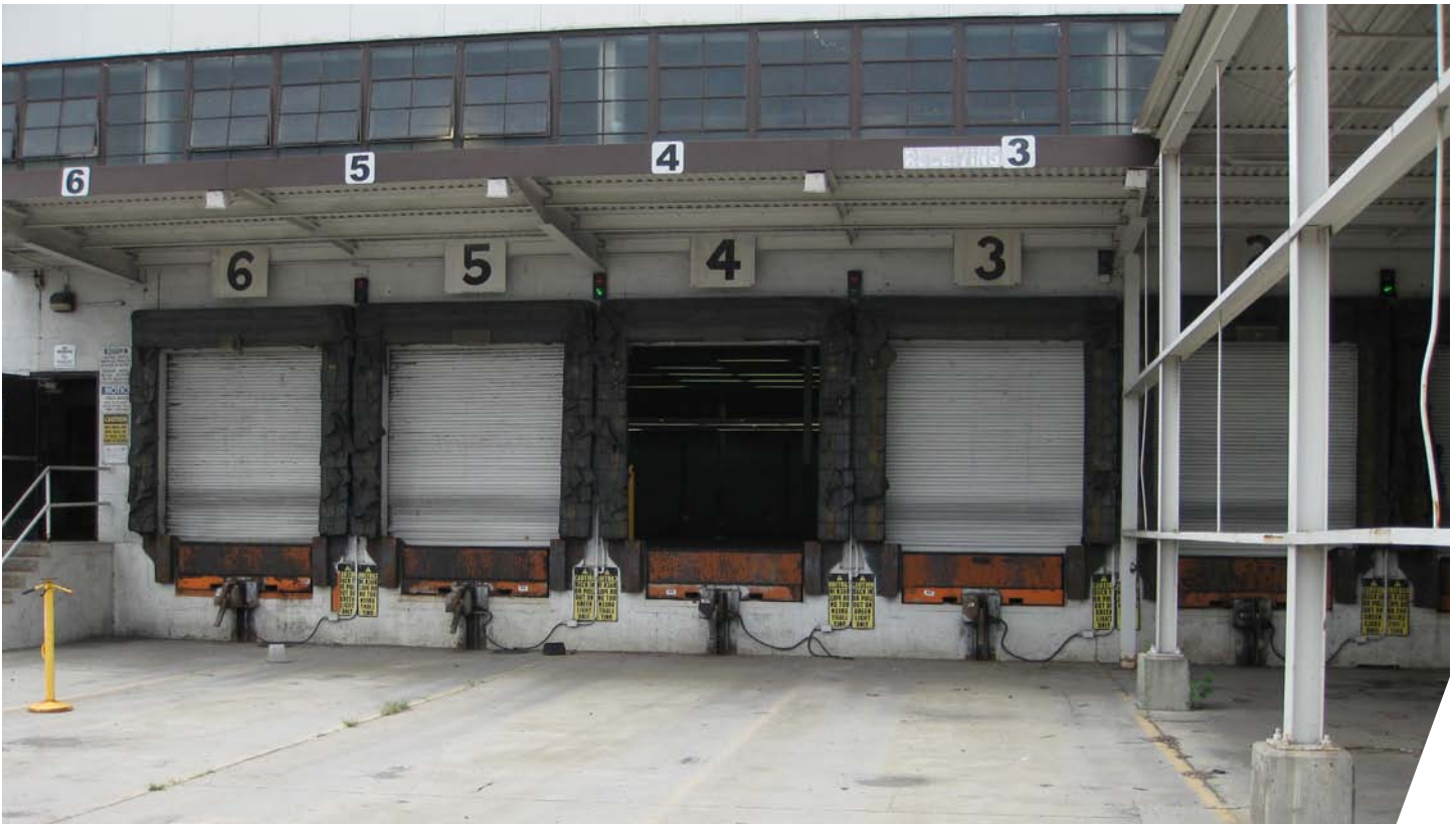
Exterior view of docks on the North side of warehouse
